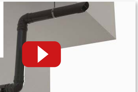
HOW TO EXTEND COAXIAL FLUE TERMINAL
